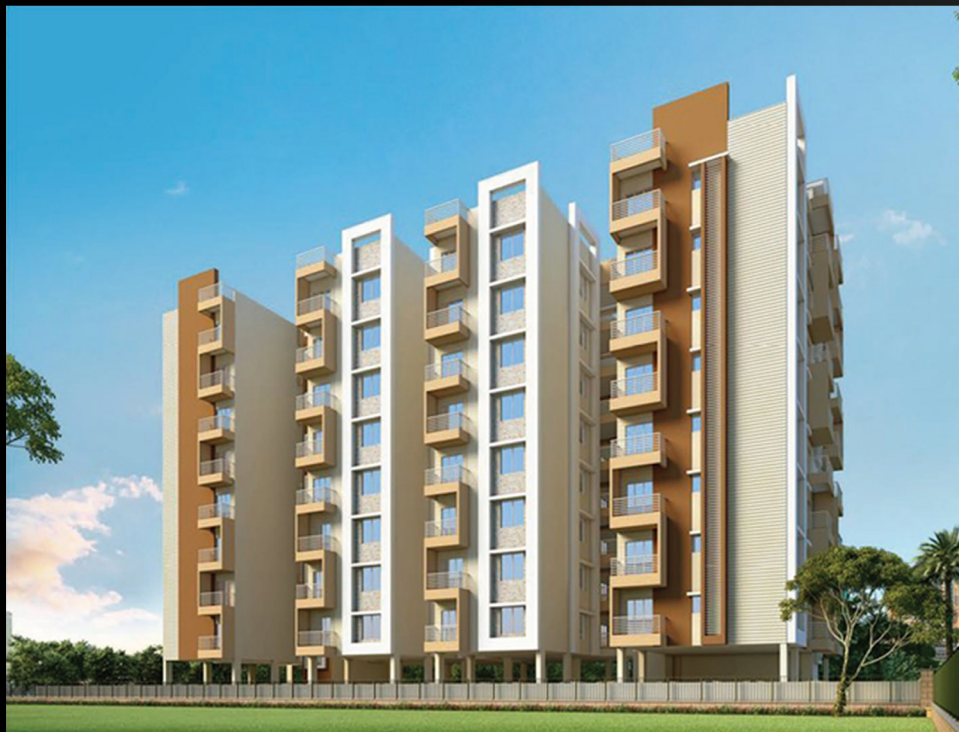
LOKHRA ROAD (G+8)
